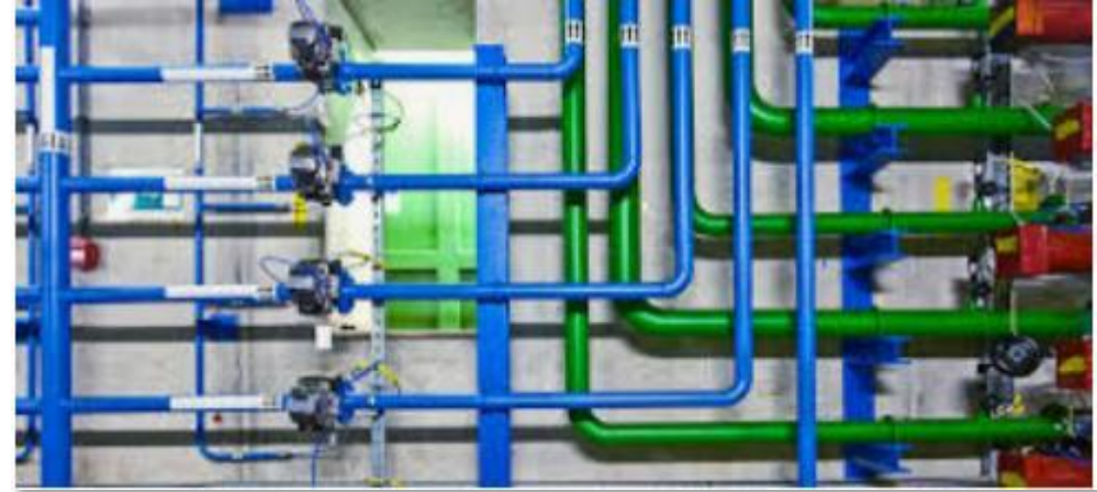
Water Meter installation for various utilities
