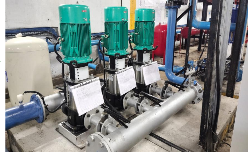
Automatic hydro pneumatic system
